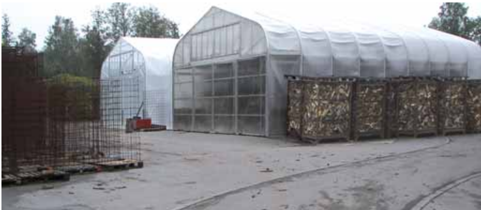
Figure 4.9.3 Greenhouses for drying log woods at the Biomassehof Allgäu (Bayern - DE)
